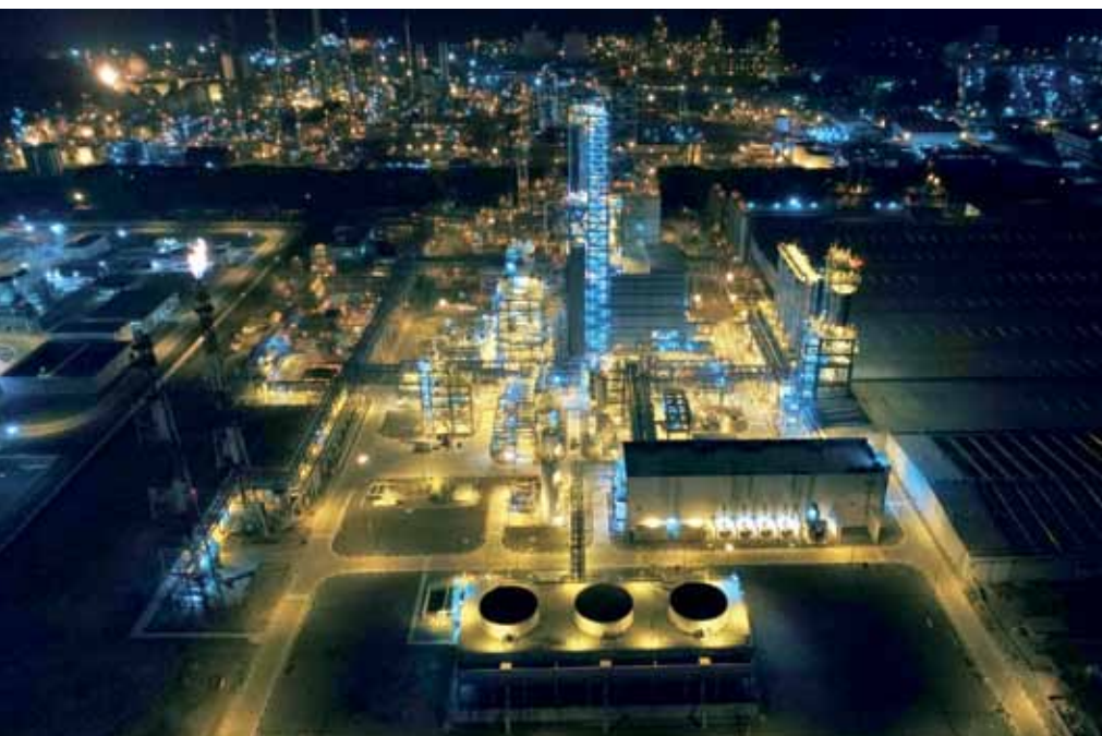
Aerial view of Chandra Asri's New Polyethylene plant.
